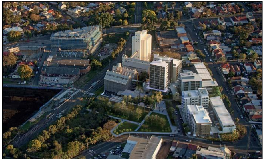
Photograph 14: A – Photomontage of former Allied Mills site at Nos. 2-32 Smith Street
