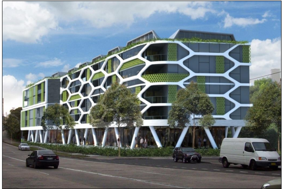
Photograph 19: E - Photomontage of Nos. 120A & 120B Old Canterbury Road Source: Tony Owen Partners
