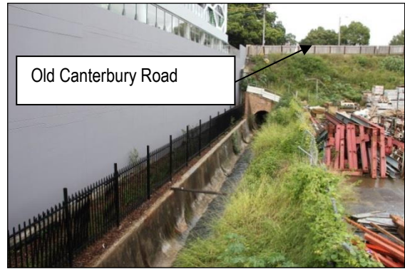
Photograph 2: The subject site looking towards the south
