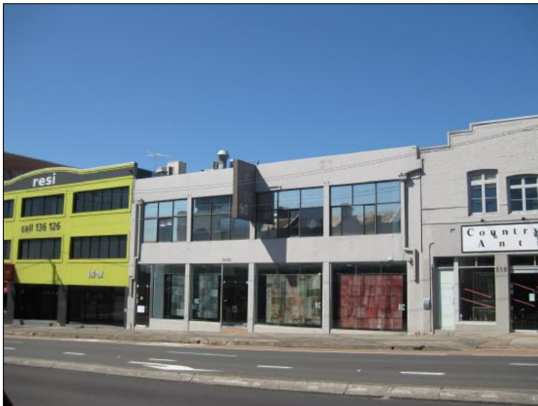
Image 1: Front elevation of existing building on the site (Parramatta Road)
