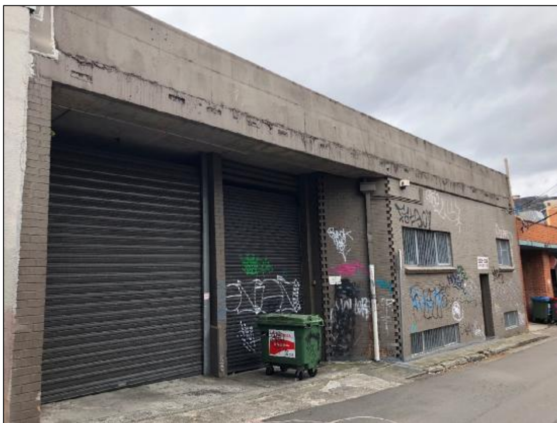
Image 2: Rear elevation of existing building on the site (Corunna Lane)
