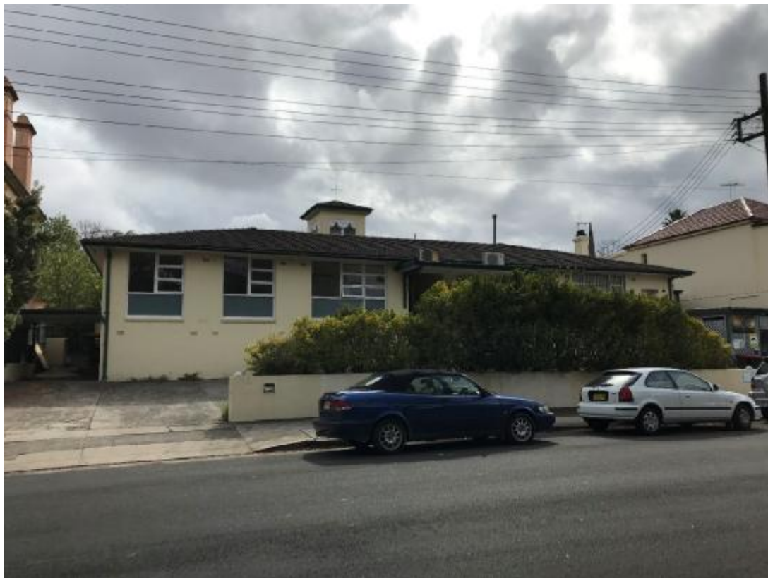
Figure 2: Site viewed from Moonbie Street.
