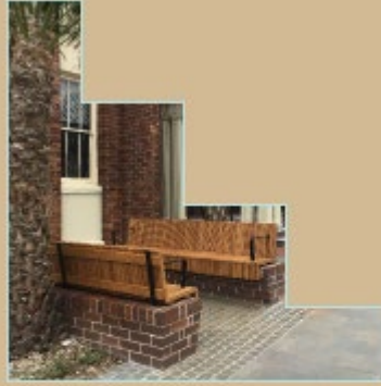
Petersham Town Hall Upgrades
