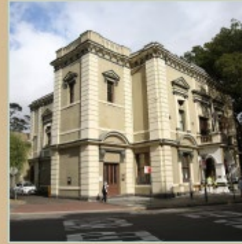
Balmain Town Hall Upgrade
