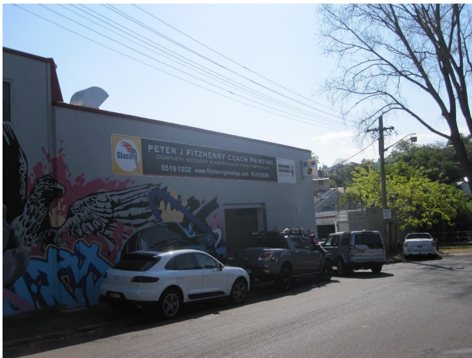
Figure 4 - Existing warehouse when viewed from Chester Street.
