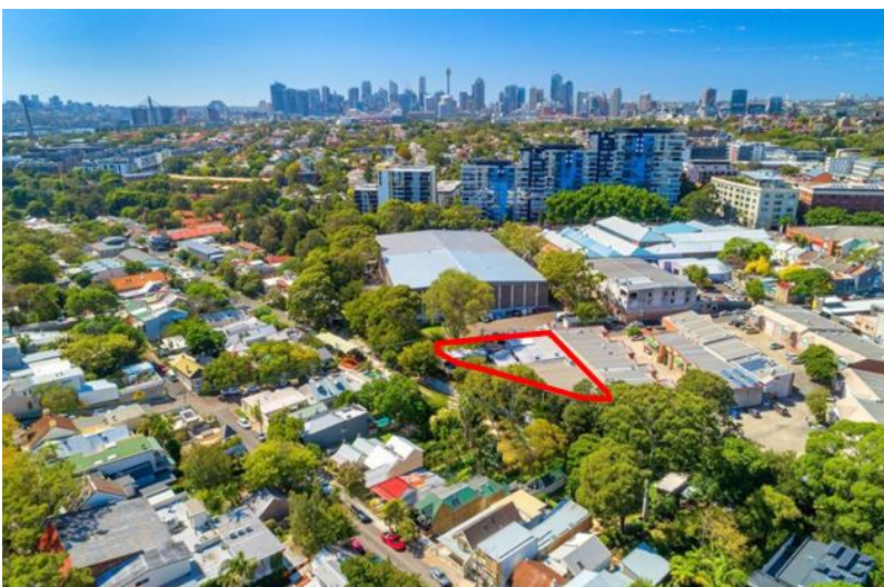
Figure 2 Aerial view of the site (shown in red) looking towards the CBD.
