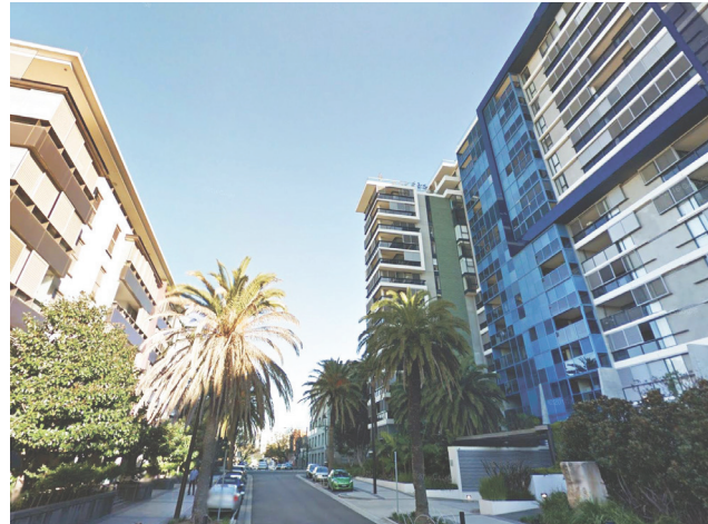
An existing high density residential development located at the corner of Booth Street and Alexandra Drive
