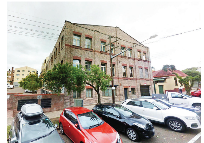
Residential flat building located near corner of Nelson Street and Collins Street
