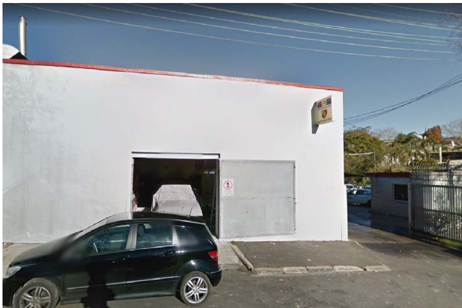
Figure 4 - Existing warehouse when viewed from Chester Street.
