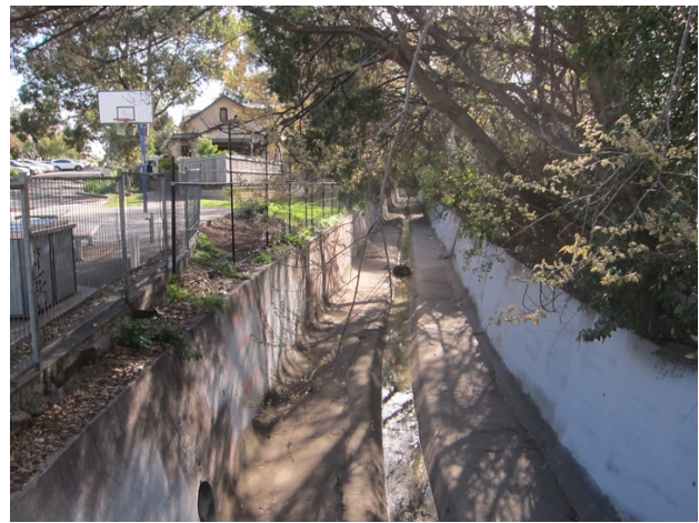
Johnstons Creek Corridor adjoining the northern side of the subject site
