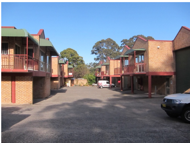
Neighbouring site: Chester Street Business Park adjoining the southern side of the subject site
