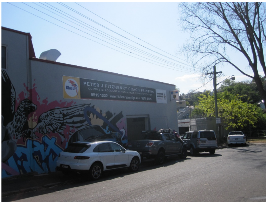
Figure 4 - Existing warehouse when viewed from Chester Street.
