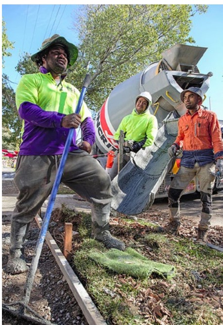
Allen Street Leichhardt footpath works in May
