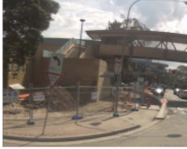
a) Finch-point at southern access to pedestrian overbridge
