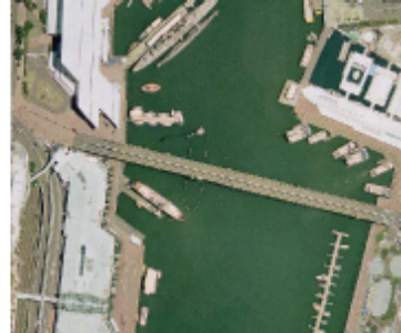
b) Straight length midway between swinging section and eastern end of bridge
