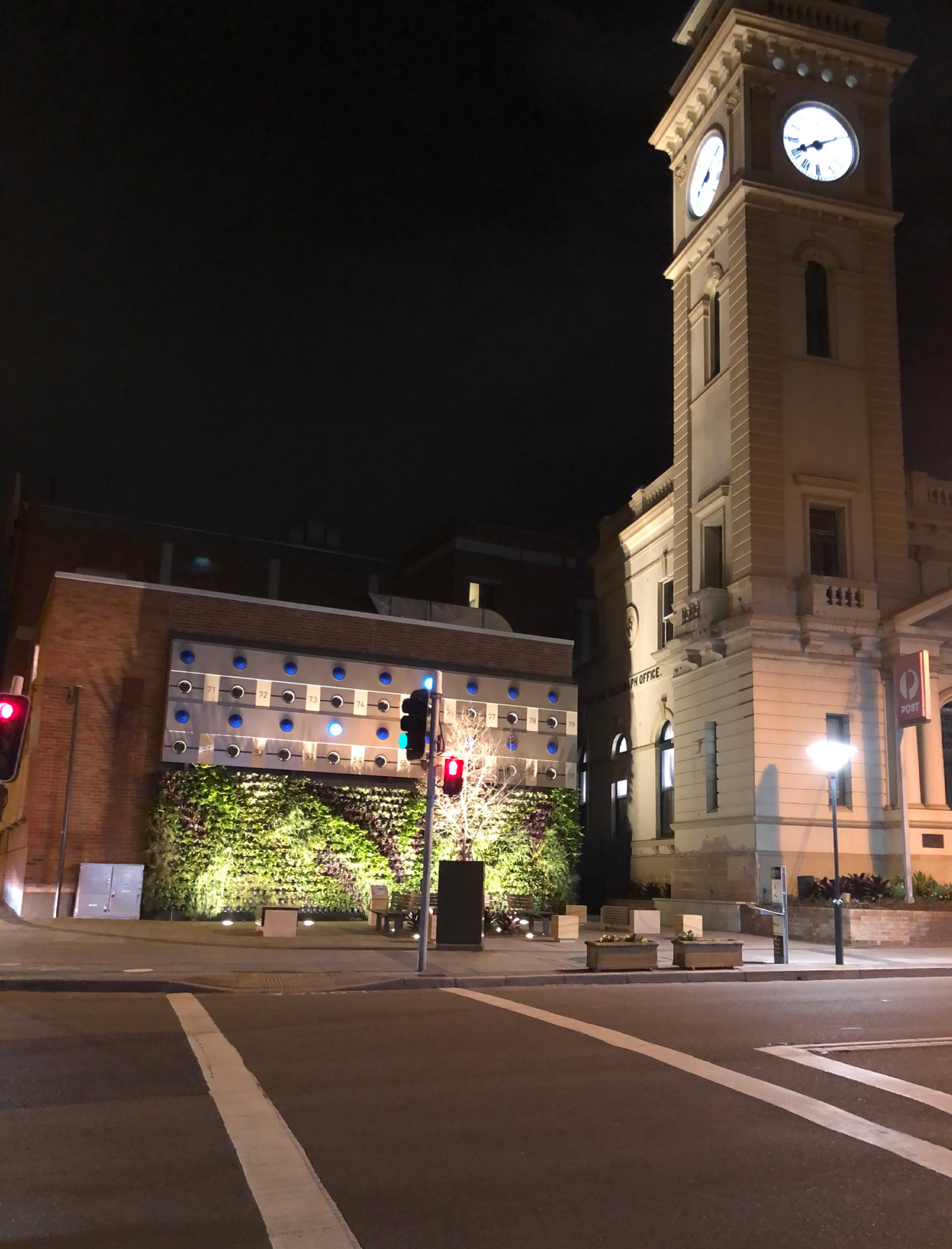
The new plaza at the former Telstra Exchange site on Darling Street Balmain was completed in July. The design includes a green wall with an artwork by local artist Sue Callanan, 'Connecting You Now', which references the telecommunications history of Balmain
