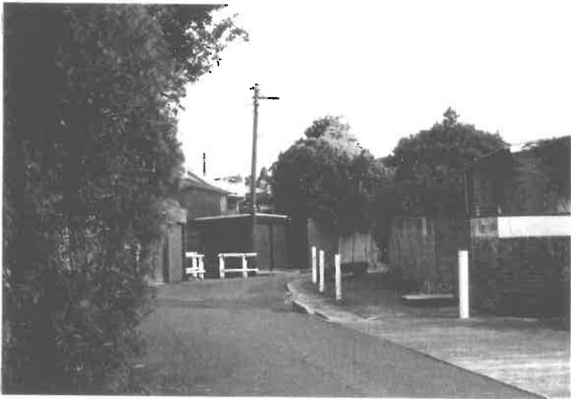
PLATE 2.3 COVERED CHANNEL, WHITES LANE
