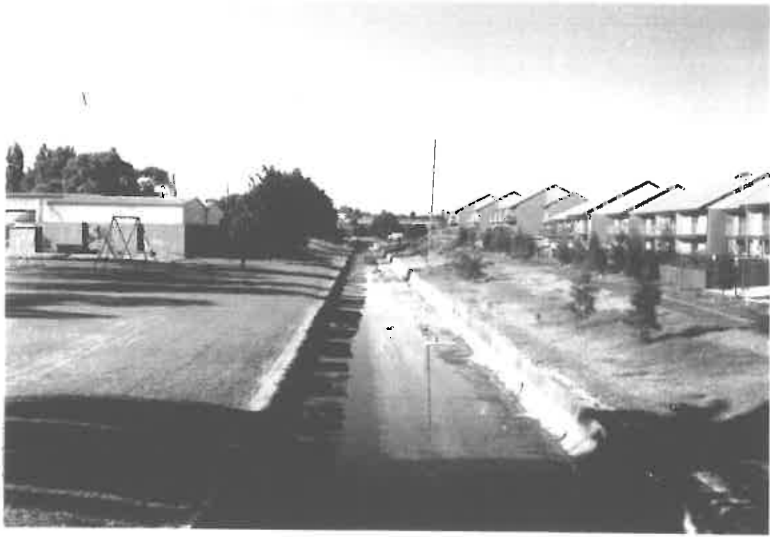
PLATE 2.1 OPEN CHANNEL NEAR DOWNSTREAM END
