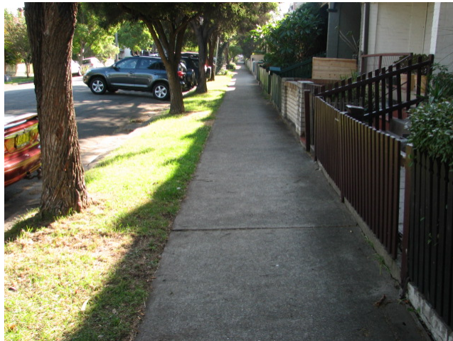
Figure 34: Verges can be converted to swales. Established trees are an issue, especially on the southern side of the street.
