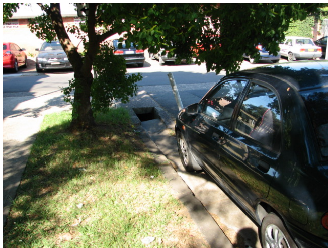
Figure 37: Gutter pits at the south west end of Goodsell St join north sloping pipes and convey water towards the railway line. There is potential for capturing and reusing this water on Camdenville Oval.
