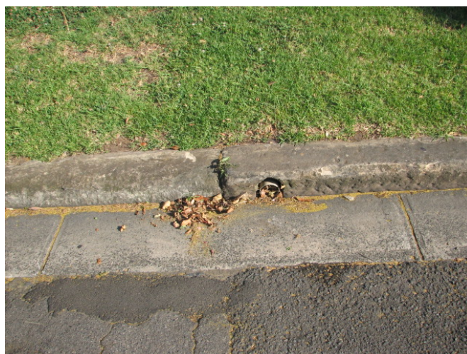
Figure 35: Runoff from homes to the street can be treated via bioretention swales established within grass verges. It would require capture of outflows which are currently conveyed to the gutter via domestic pipes.
