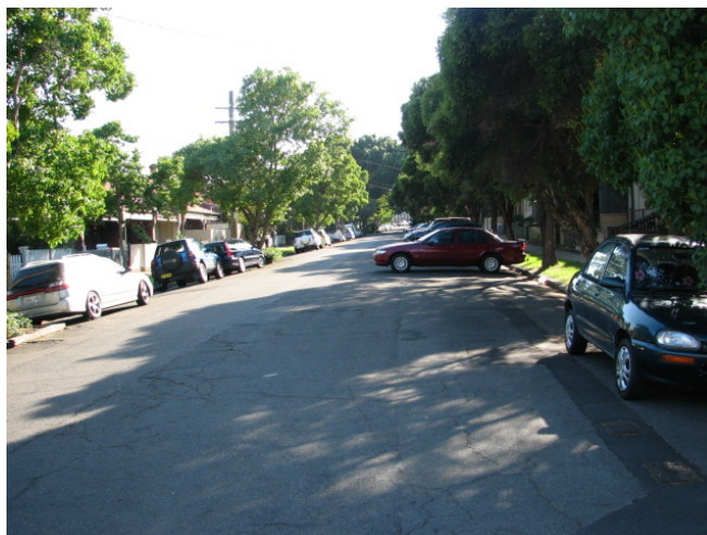
Figure 18: Much of Goodsell St has a mix of parallel and perpendicular parking. The grassed verges offer opportunity for WSUD features.
