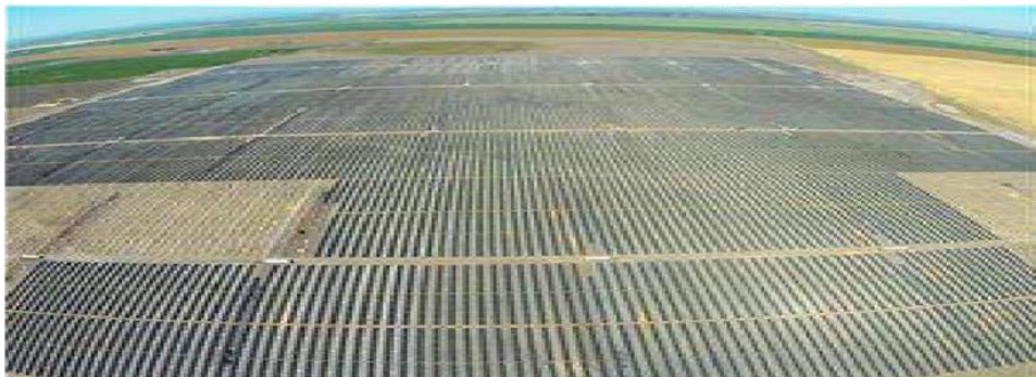
Figure 3: Moree solar farm
