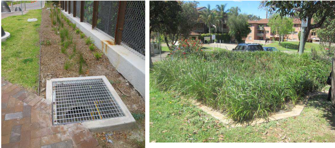
Figure 18 Steel edge (left) and concrete edge (right)
