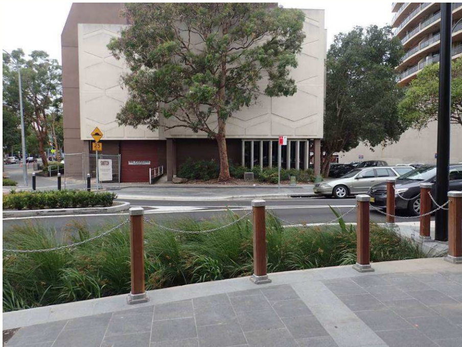
Figure 24 Chain and bollard fencing
