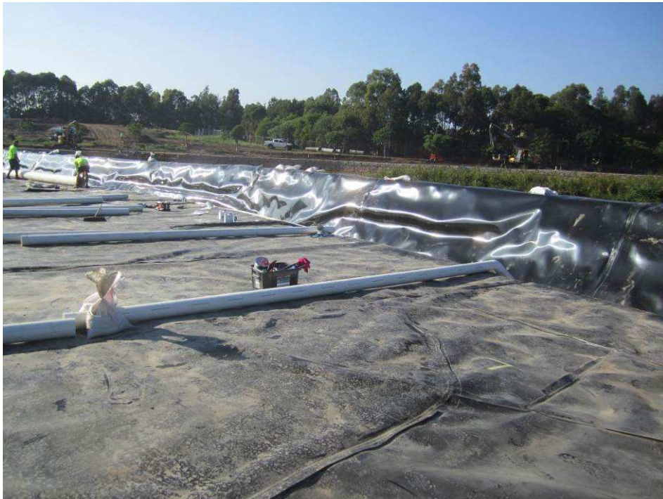
Figure 28 Subsoil drains being installed on top of a HDPE liner
