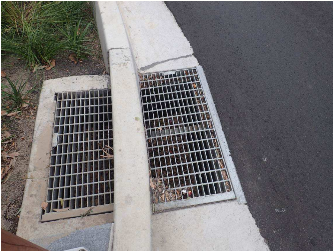
Figure 12 Double pit arrangements in streetscape rain garden
