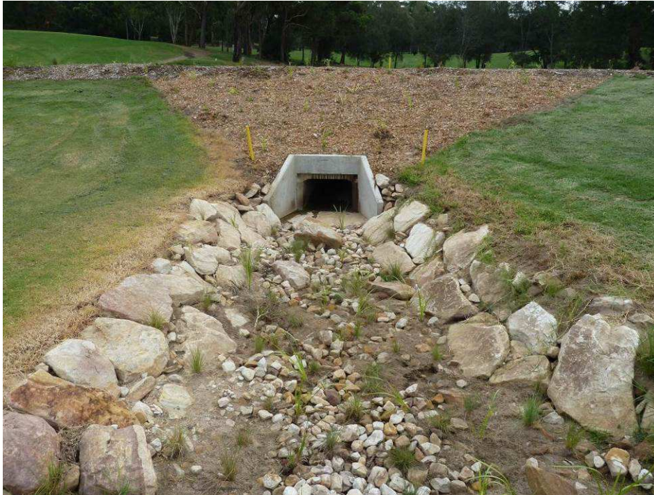
Figure 11 Irregular rock scour pad – not recommended due to difficulty of cleaning out sediment
