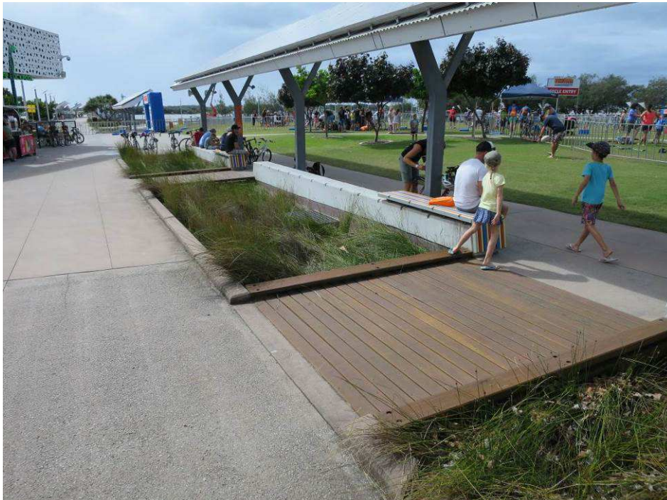
Figure 20 Low kerb wheel stop barrier edge (left) and seating wall edge (right)
