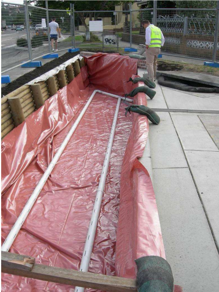
Figure 26 Bricks plastic liner and sub soil drains
