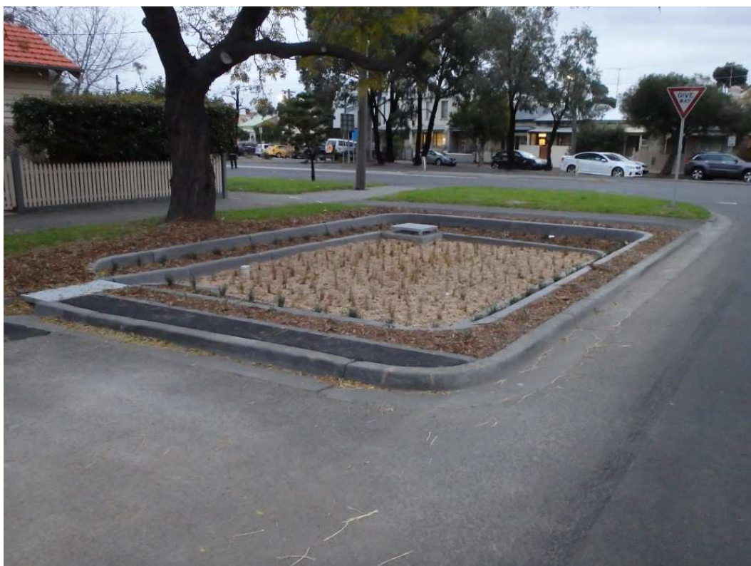
Figure 19 Planted buffer strip around rain garden with low kerb walling
