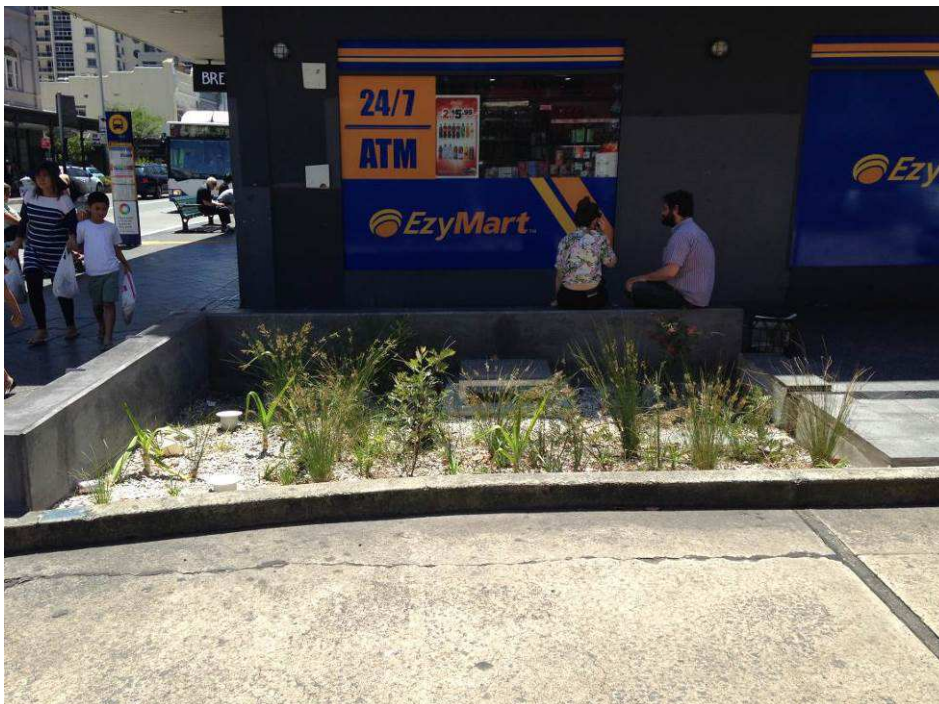
Figure 21 Kerb edge (foreground), raised paver edge (right hand side) and seating wall edge (background) to a rain garden.
