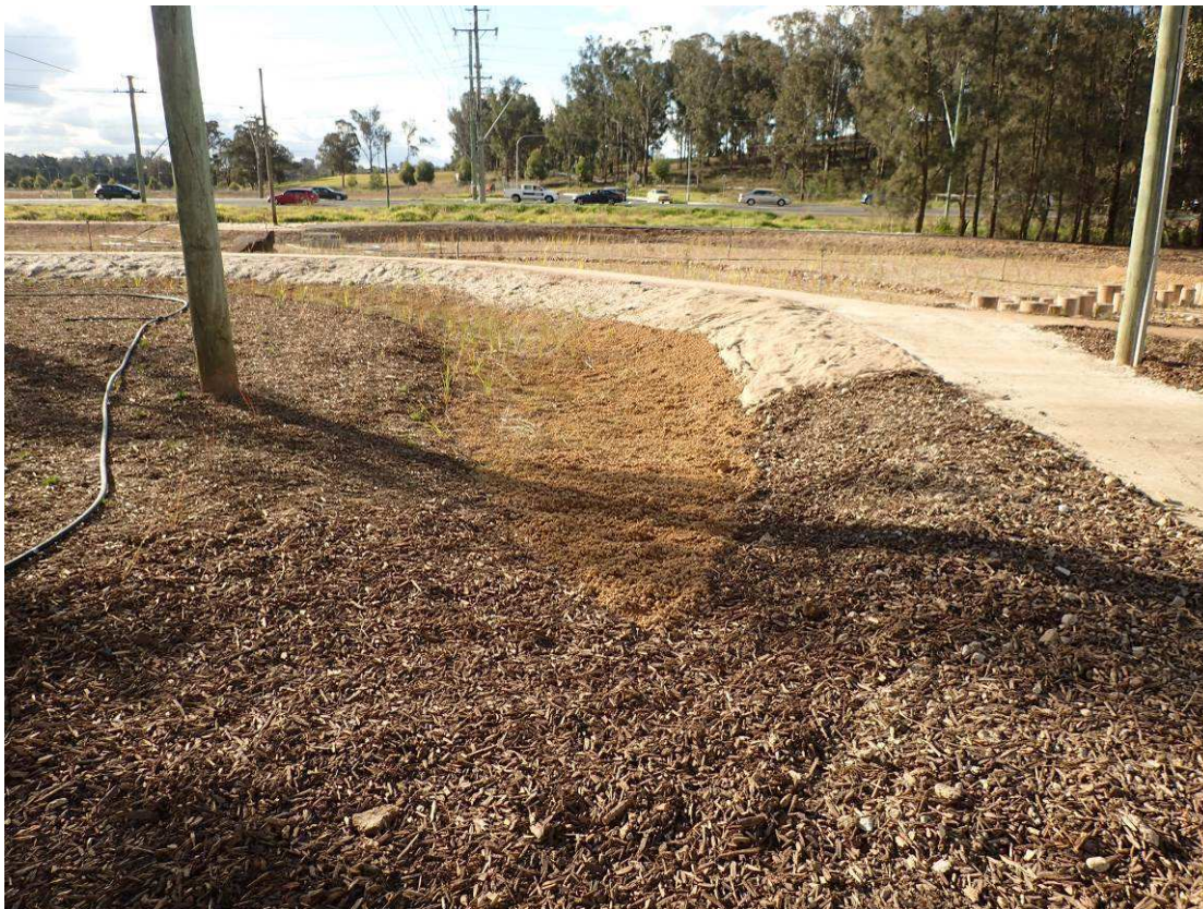
Figure 16 Bark mulch surrounding rain garden with jute covering bark mulch on batters outside of ponding area and sandstone rock mulch on base
