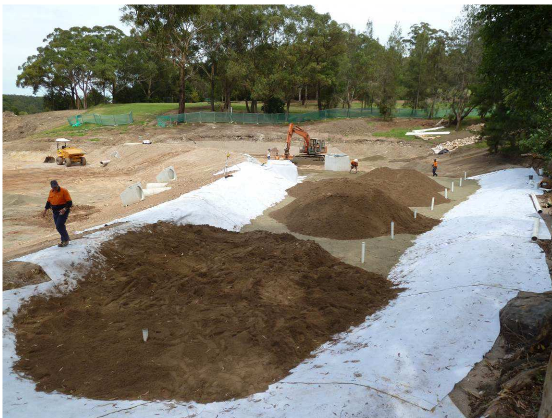
Figure 5 Rain garden media overlying glass sand and a geosynthetic clay liner
