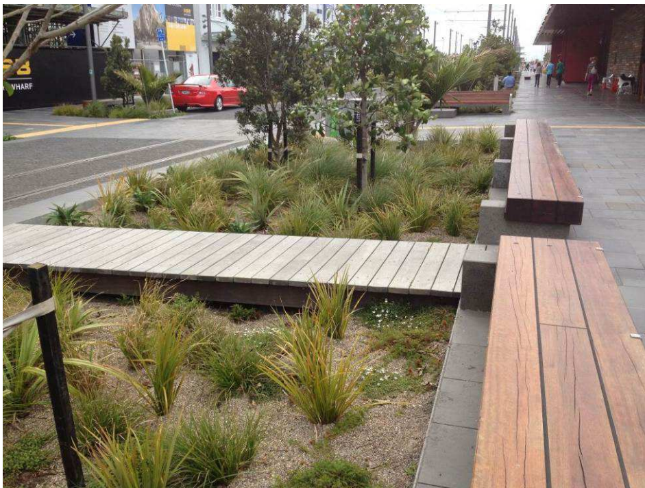
Figure 23 Street furniture (seating on right) used as an edge to the rain garden
