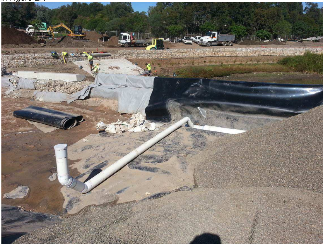
Figure 27 Flushing point connected to a subsoil drain prior to back fill
