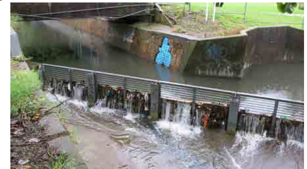
Western Channel trash rack on the Cooks River
