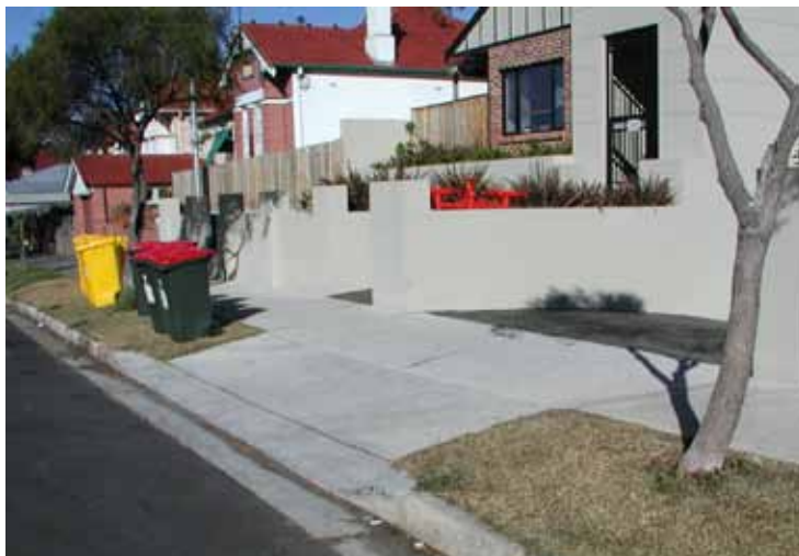
Hard surfaces increase the volume and speed of stormwater runoff that carries pollutants to the Cooks River.
