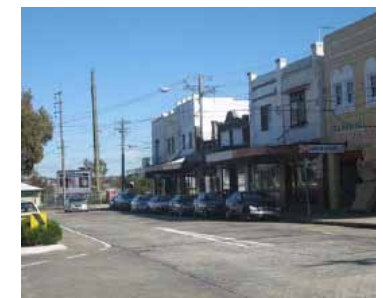
Shops at Dulwich Hill Station along Wardell Road.
