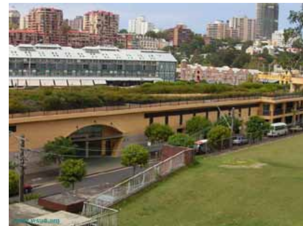
WSUD at Wharf 11 in Sydney includes a vegetated roof that has the multiple benefits of filtering rainwater, cooling the building and providing habitat. (Photo WSUD.org).
