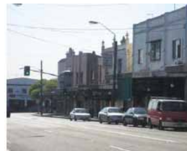
Dulwich Hill Shops, New Canterbury Road.
