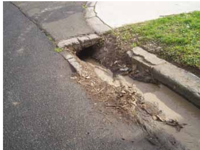
Sediment escaping from building sites enters into the stormwater system that discharges to the Cooks River.
