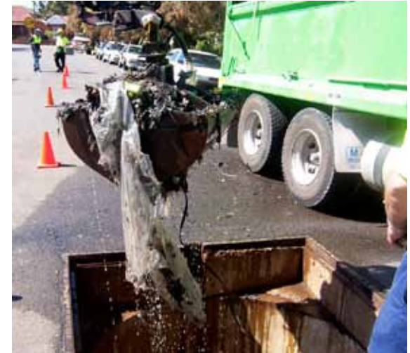
Cleaning out the CDS unit in Balfour Street that traps some gross pollutants heading for the Cooks River.
