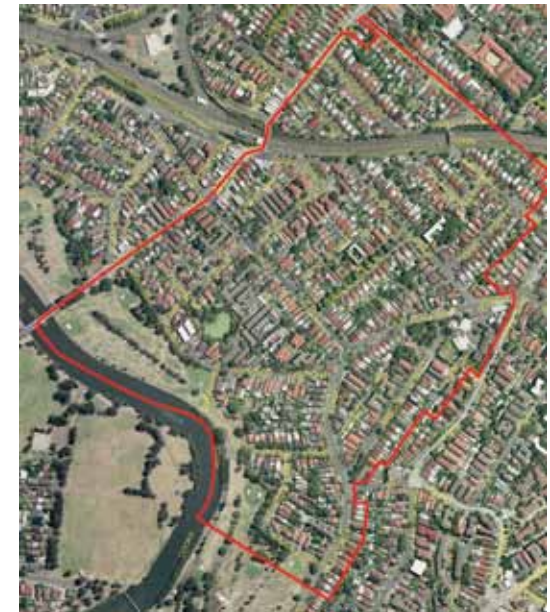
Riverside Crescent Subcatchment aerial view, 2007.
