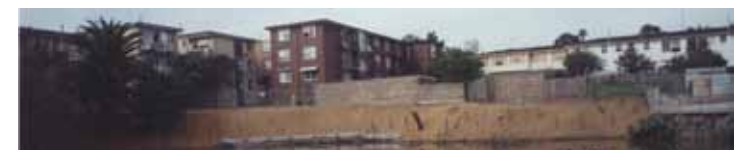
Environmental restoration works, 1993.
