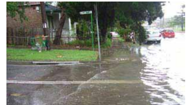
Localised flooding on Illawarra Rd, February 2008. Photo by Paul King.
