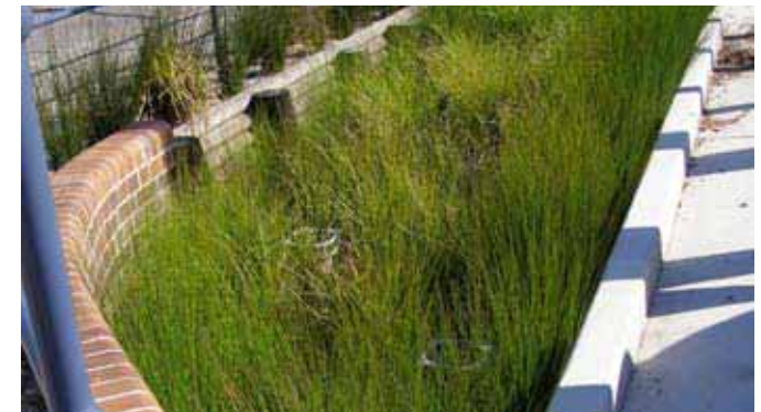
Hill Street rain gardens built in October 2007 as a result of the Illawarra Road Subcatchment Planning. Photos April 2008.
