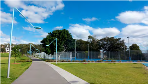
Off-road concrete path (Prince Alfred Park - note that this path is 5 m wide)
