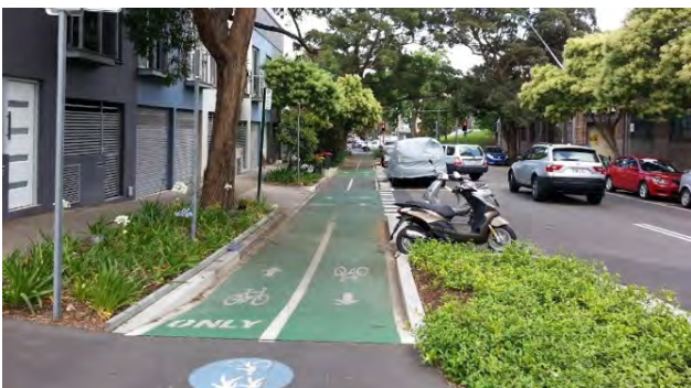
On-road bidirectional separated cycleway (typical City of Sydney separated cycleway)
