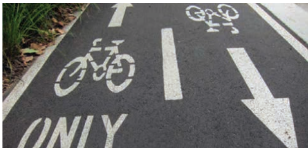
Separated cycleways are typically indicated with bike signs and arrows. (City of Sydney)
