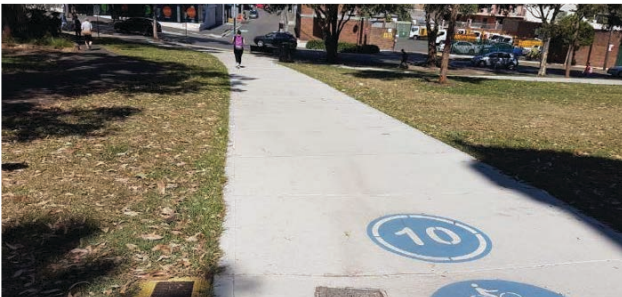
Redfern secondary shared path
