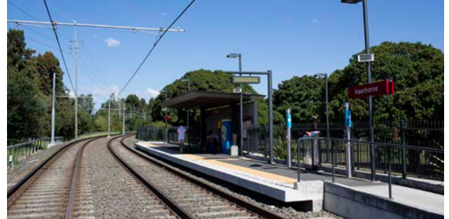
Hawthorne light rail station
