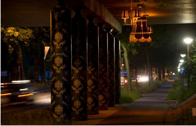
Underpass Activation under bridge
